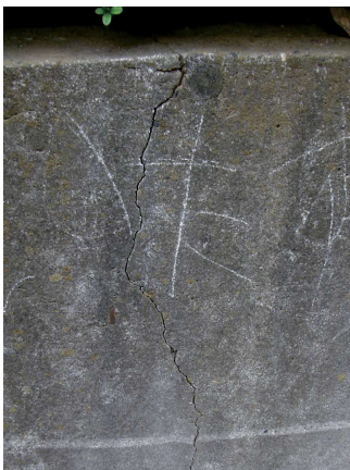
Photo 1. Crack of a Concrete Retaining Wall (No.23 in Sampling Point ⑤)
