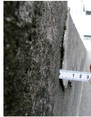
Photo 2. Narrow Gap of an Old Concrete Wall (No.29 in Sampling Point ⑥)
