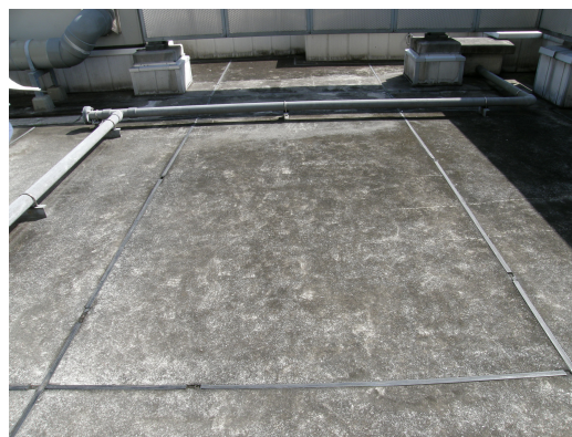
Photo 1. Researched Roof of a Five-Story Building
